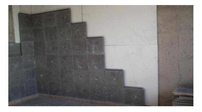
A typical concrete wall installation, over Calcium silicate board. Note: Calcium silicate board is not necessary with "Hybrid" tile install.
